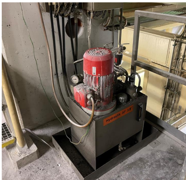
Figure 14: Hydraulic system from the airfoil system
